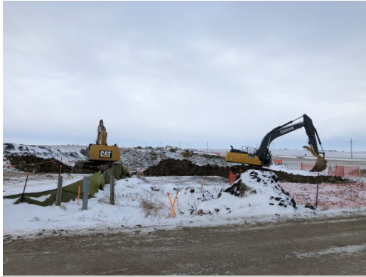
SF 43A, photo facing west, excavators and one dozer moving dirt.
