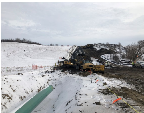
SF 39, photo facing east, equipment digging out creek crossing.
