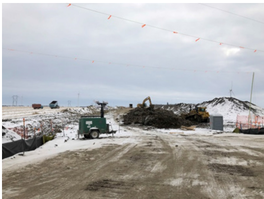
SF 45, photo facing east, one dozer and one excavator pushing dirt on the ROW.
