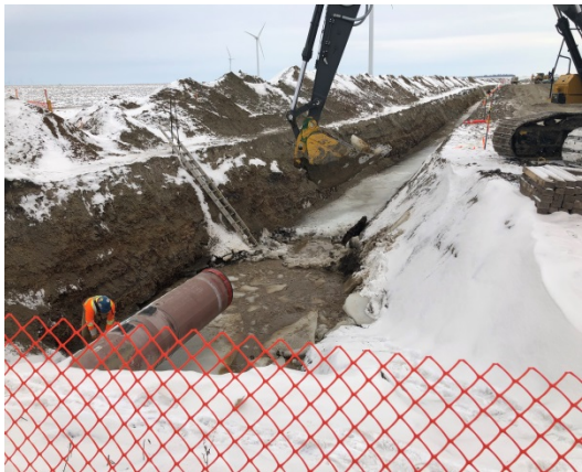
SF 49, photo facing east, excavator removing ice from trench.
