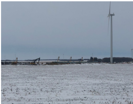
SF 48, photo facing west, side booms lowering in pipe.
