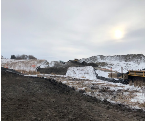
SF 40, photo facing east, one dozer pushing dirt up hill.
